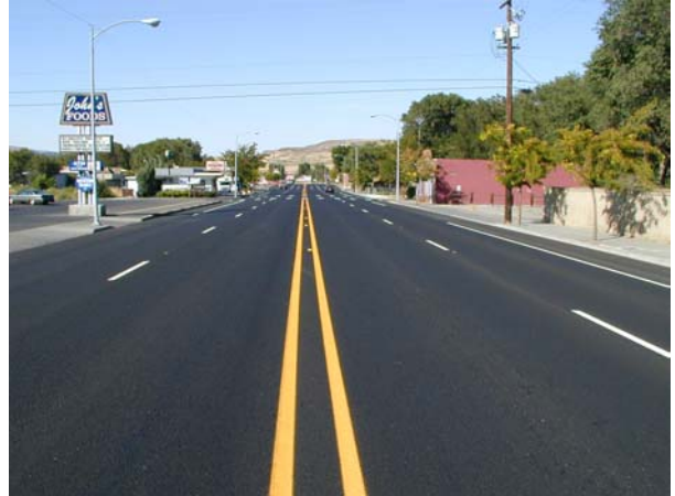
Photo 23. Soap Lake – Final NovaChip® surface.
