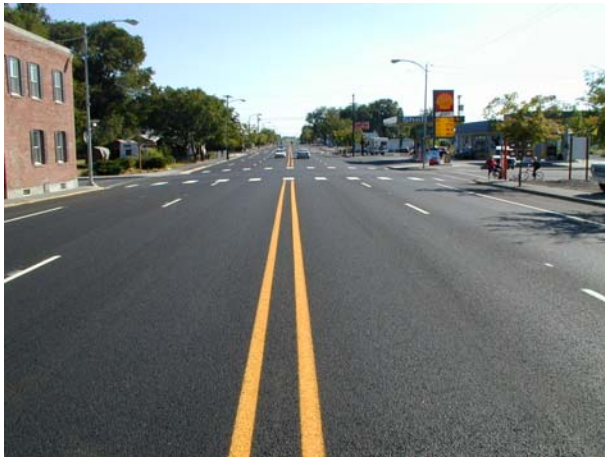
Photo 24. Soap Lake – Final NovaChip® surface.
