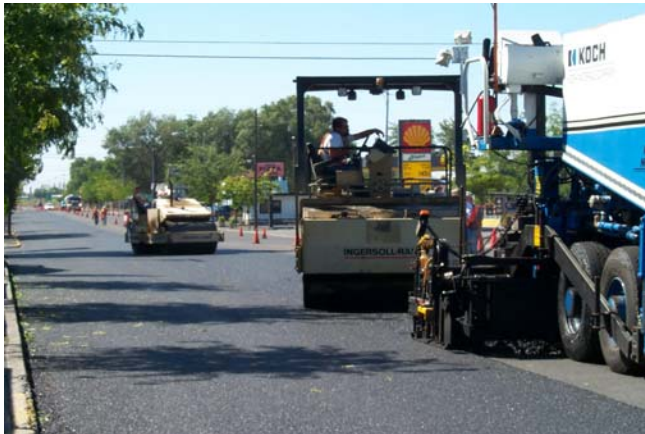
Photo 15. Rolling (seating) the NovaChip® surface.
