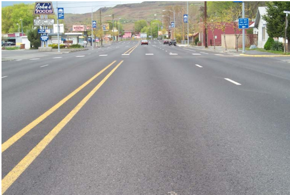
Photo 26. NovaChip® overlay through Soap Lake – May 2003.
