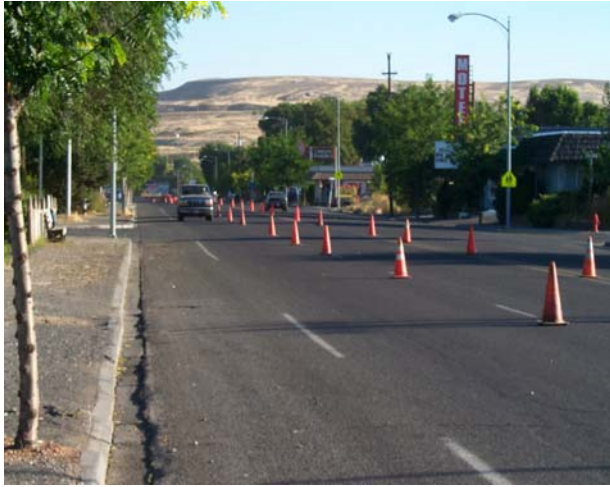
Photo 13. Traffic control in place.
