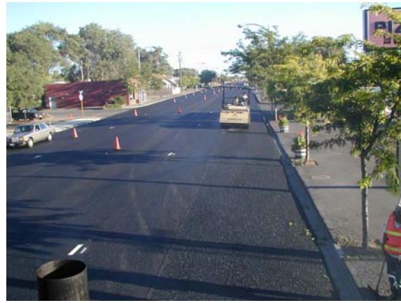
Photo 16. Compaction of the NovaChip® roadway surface.
