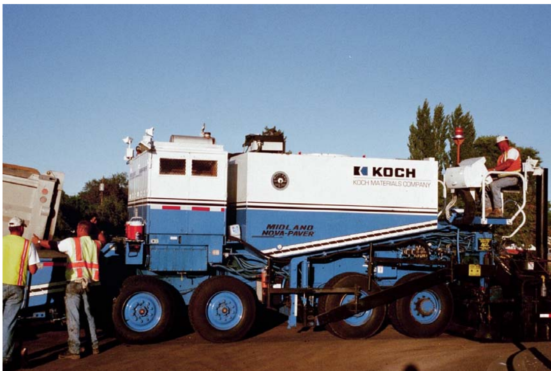
Photo 1. Novachip Paving Machine.
