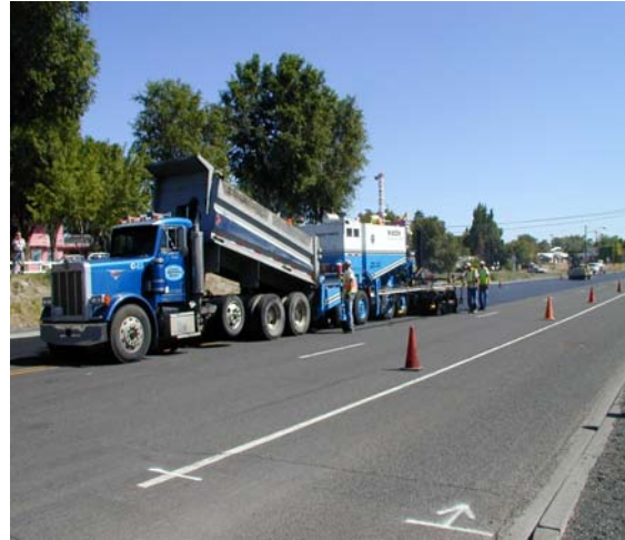
Photo 14. NovaChip® paving operation.
