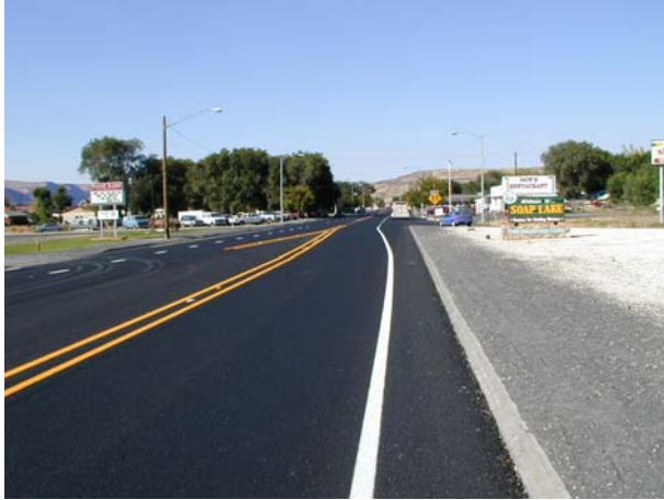
Photo 22. Soap Lake – Final NovaChip® surface.
