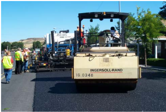
Photo 20. Rolling directly behind the NovaChip® paver with a 15 ton roller.
