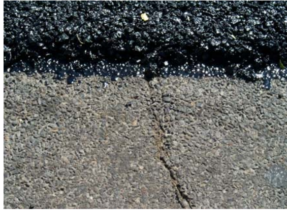
Photo 8. NovaChip® asphalt placed over existing transverse cracks.
