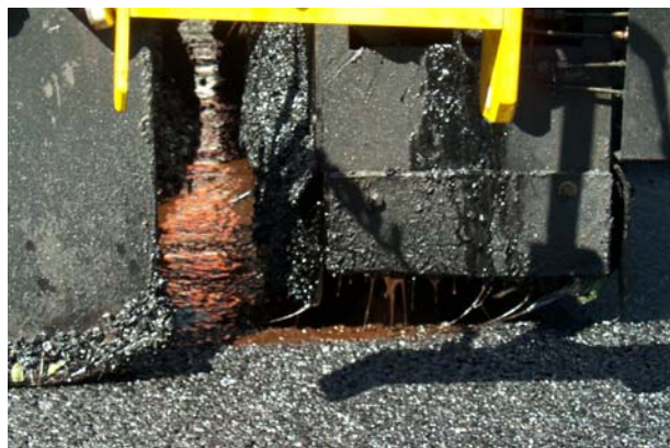
Photo 17. Novabond® Membrane being applied prior to the hot mix asphalt.
