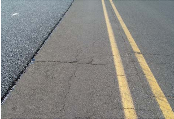
Photo 7. NovaChip® placed over existing roadway. (The existing low severity cracks were not sealed.)
