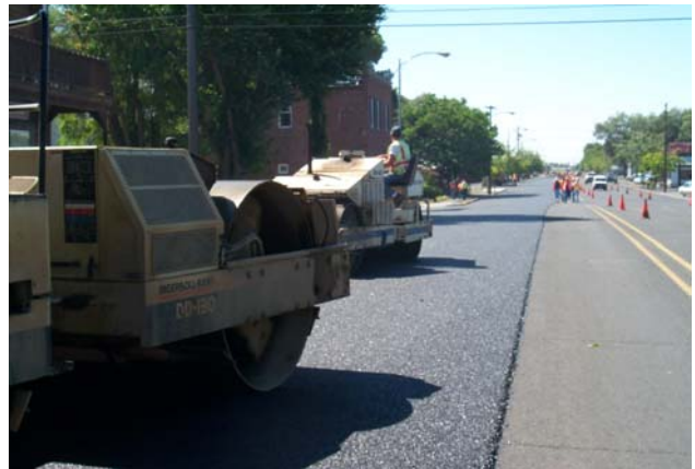
Photo 21. Compaction was completed with a 15 ton breakdown roller and 12 ton finish roller.
