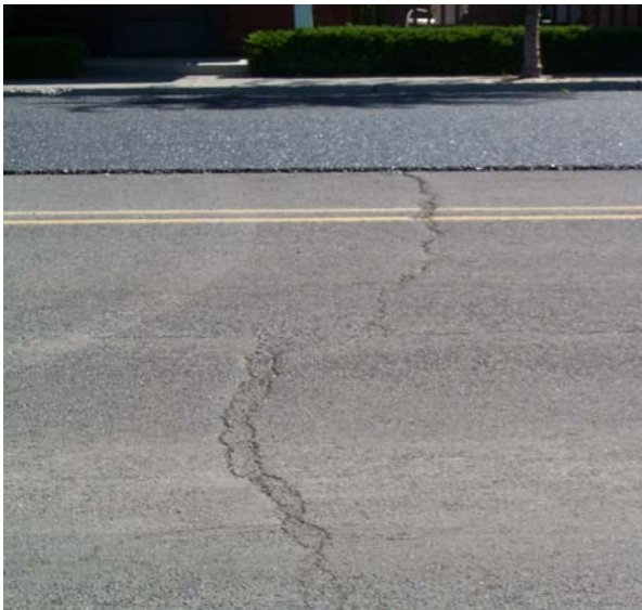
Photo 9. NovaChip® placed over an existing transverse crack (high severity).
