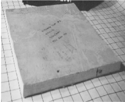
a) Category A - No Visible Damage
