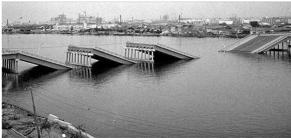
Figure 3.4. Showa River bridge following 1964 Niigata earthquake.
