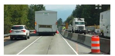
Oversized truck freight example; modular home straddling both lanes on Interstate 90 at a bridge rehabilitation work zone with a reduced traveled way.
