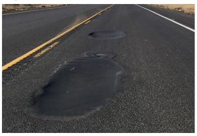
This distress typically results in full-depth repairs although a partial-depth patch or a micro-grind may be used depending on the cause of the distress.
