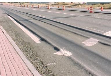
There are a few options available to address this type of roadway distress. Rut filling with HMA is the most widely used, however; a second rut filling option is to utilize chip seal materials. Grinding of rutting can also occur but care must be taken to ensure this option will remove ruts until preservation occurs.
