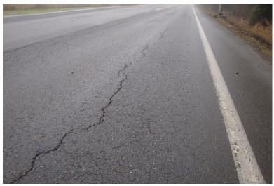
This type of crack is usually a non-working crack that can be treated with a crack sealing material. It is highly recommended that these cracks are filled before getting to a width greater than a  $\frac{1}{2}$  inch to reduce sealant cost. Although this is the most cost-effective treatment option available, attempting to seal cracks that are greater than  $\frac{3}{4}$  inch is not recommended.
