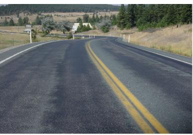
Removal and replacement of flushed or bleeding pavement areas is an expensive, but sometimes cost-effective method of repair. Another option is to perform a chip seal with minimal or no emulsion but this approach necessitates proper prior planning. If repairs are not possible prior to a seasonally wet period, contact the regional traffic engineer to evaluate friction and the need for posting "Slippery When Wet" signs.
