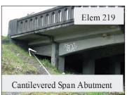
The definition, condition evaluation, and units are the same as for the WSDOT element 200 where this element is defined as the soil retained behind the abutment and wing walls or retaining walls that support an asphalt roadway or approach slab. The fill evaluation should not extend beyond 25 feet or the approach slab, whichever is greater. Erosion outside of the abutment/wingwalls can be documented in the notes, but is not included in the evaluation of the element condition states.
