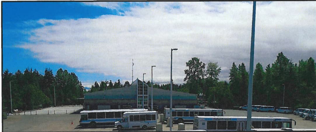
CTS Maintenance Yard and Shop Facility
