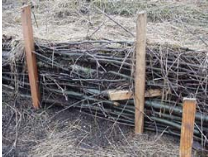
Figure 740.12 Willow Fencing With Brushlayer (brushlayer is hidden below soil from construction).
