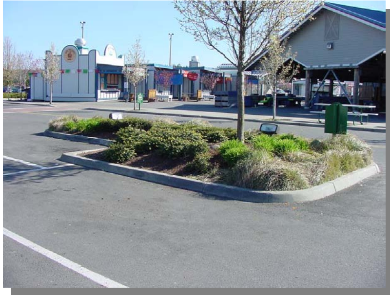
Figure 630.11 Raised curbs around end island
