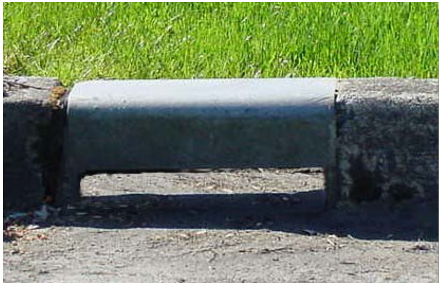
Figure 630.6 Curb interruption to facilitate drainage into bioswale
