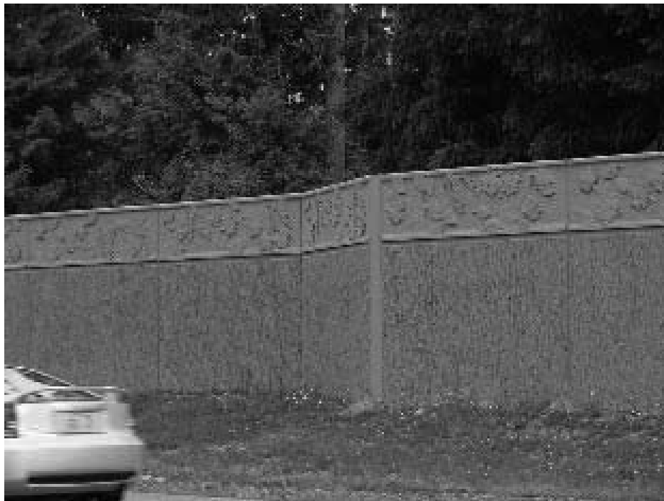
Figure 910.1 Noise wall enhancement in Mill Creek
