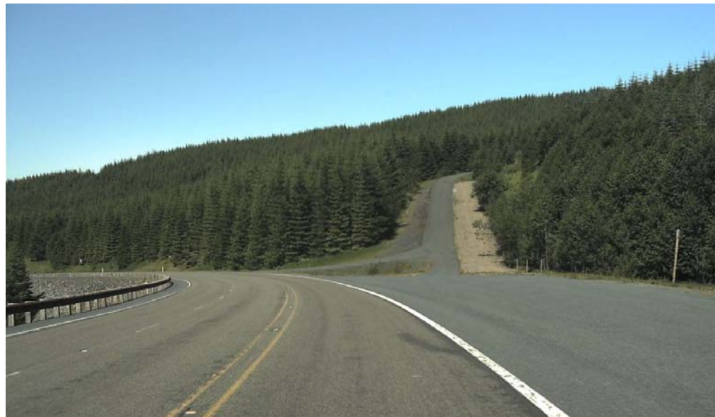
Emergency Escape Ramp Example Exhibit 1270-10
