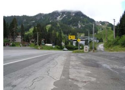
Key View 2 – View of Pedestrian Bridge from Parking Lot on North Side of US 2 at Mile Post 64.62
