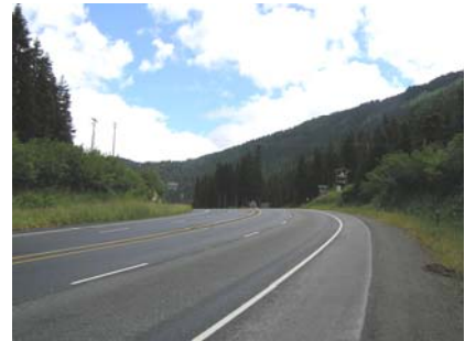
Key View 3 – View East toward the Proposed Bridge from the Shoulder of US 2 at Mile Post 64.50
