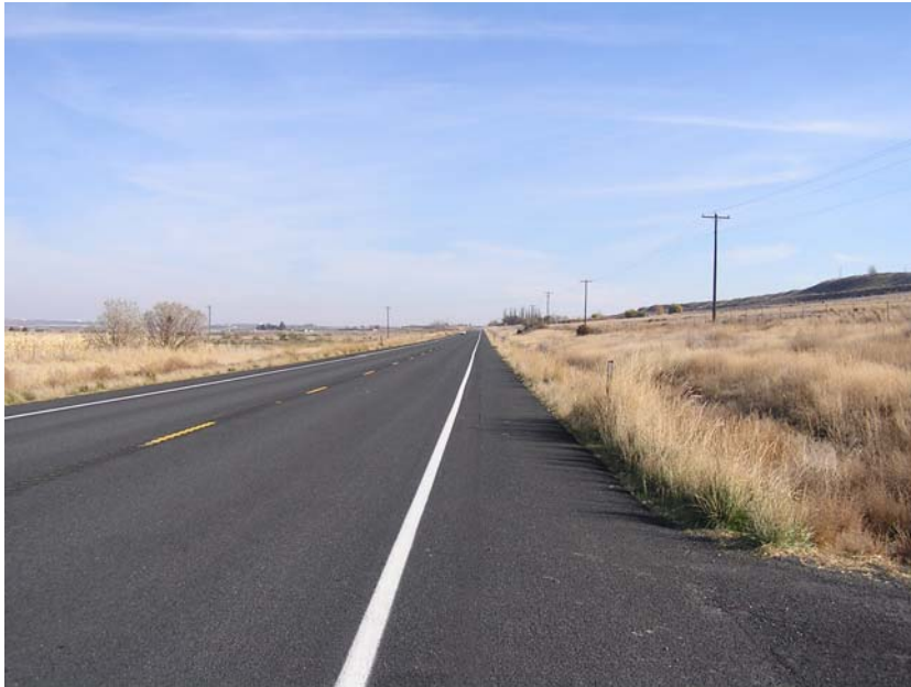
Exhibit 3-2 Key View 1 - View towards project – MP 34.87
