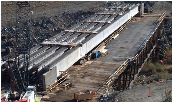
In 2016, Douglas County used federal and state funding to replace a damaged timber bridge on SR 173 over Foster Creek with a prestressed concrete girder bridge for increased stability.
