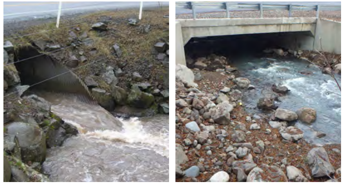
WSDOT's new culvert (right) on State Route 129 allows fish to access habitat upstream of the old barrier (left) on Rattlesnake Creek.
