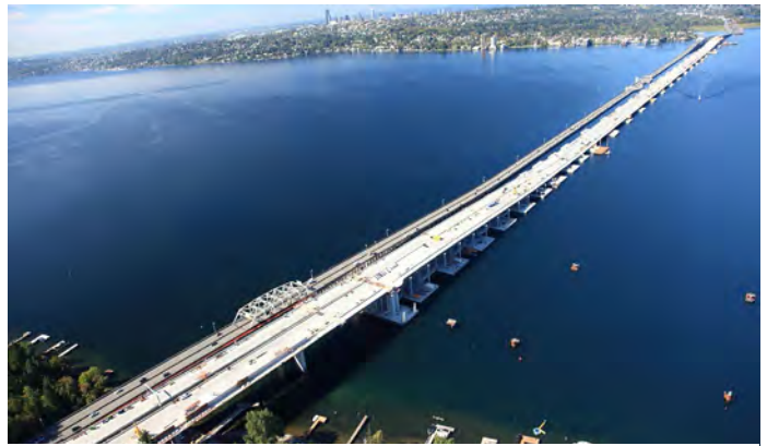
The old SR 520 bridge was WSDOT's longest structurally deficient bridge, totaling 7,518 feet long (442,810 square feet of deck area). A new floating bridge was opened to traffic in April 2016.
