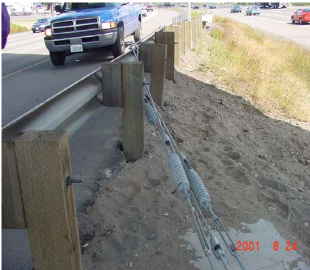
FIGURE 3 Washington State cable barrier transition to W-beam guardrail
