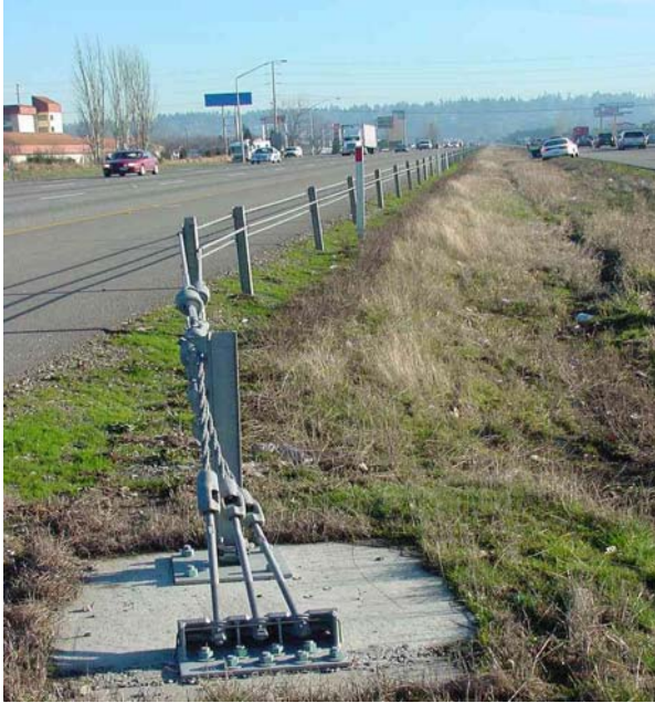
FIGURE 2 Washington State cable barrier terminal
