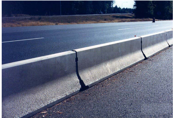
FIGURE 1 Typical precast barrier installation-
