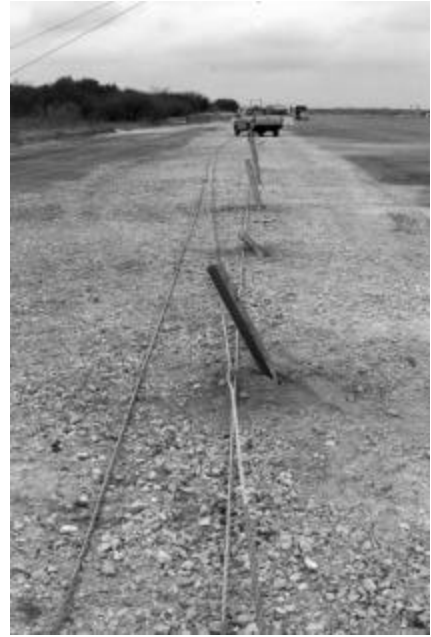
FIGURE 7 Barrier damage from pickup truck test.
