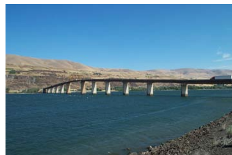
U.S. 97 Biggs Rapids Bridge near Goldendale (Source: WSDOT Bridge Office)
