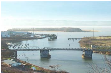
U.S. 101 Simpson Avenue Hoquiam River Bridge (Source: WSDOT Bridge Office)
