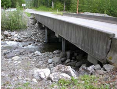
SR 542 Boulder Creek Bridge near Glacier (Source: WSDOT Bridge Office)
