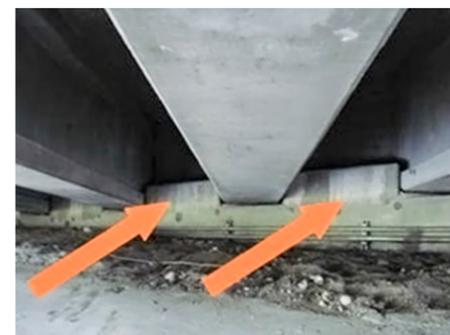
Girder stops are blocks of reinforced concrete that are installed between girders at the abutments and intermediate piers. The girder stops prevent the girders from sliding sideways on the abutment/pier.
