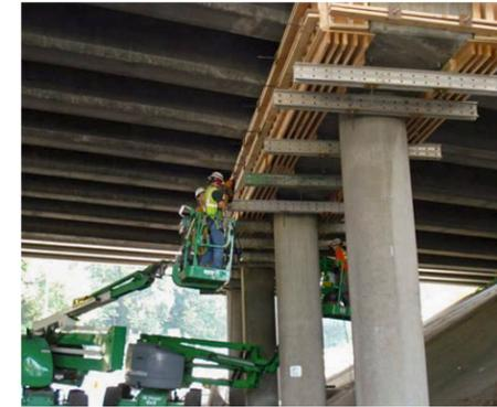
Crossbeam bolsters consist of adding reinforced concrete to the sides of existing crossbeams (the beam that sits on top of the columns). The purpose of these bolsters is to increase the crossbeam shear and moment capacity...As well as to increase the seat width... so girders don't fall off the crossbeam.
