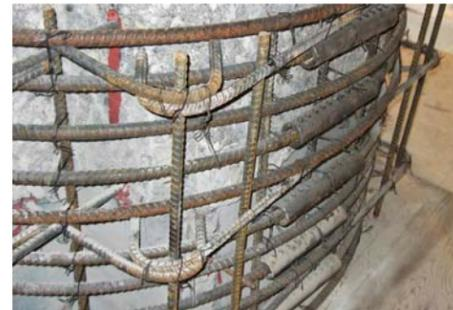
This is what a column looks like when we "wrap" it with rebar to help stabilize the concrete. The concrete may crack, but the new reinforcing steel will keep the concrete from turning to rubble and falling out.
