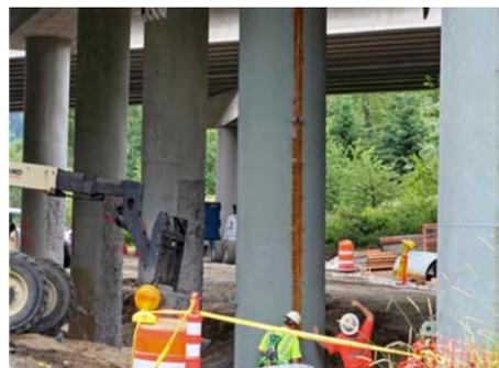
Columns (as shown above) are being wrapped with a steel jacket to contain and stabilize the concrete column which prevents cracking and possible failure during an earthquake.
