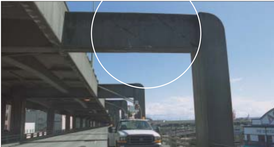
Top: Alaskan Way Viaduct from the south in Seattle Above: Cracking on viaduct support beams
