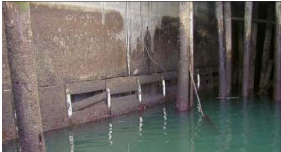
Above: Holes in the Seawall sheet pile wall
