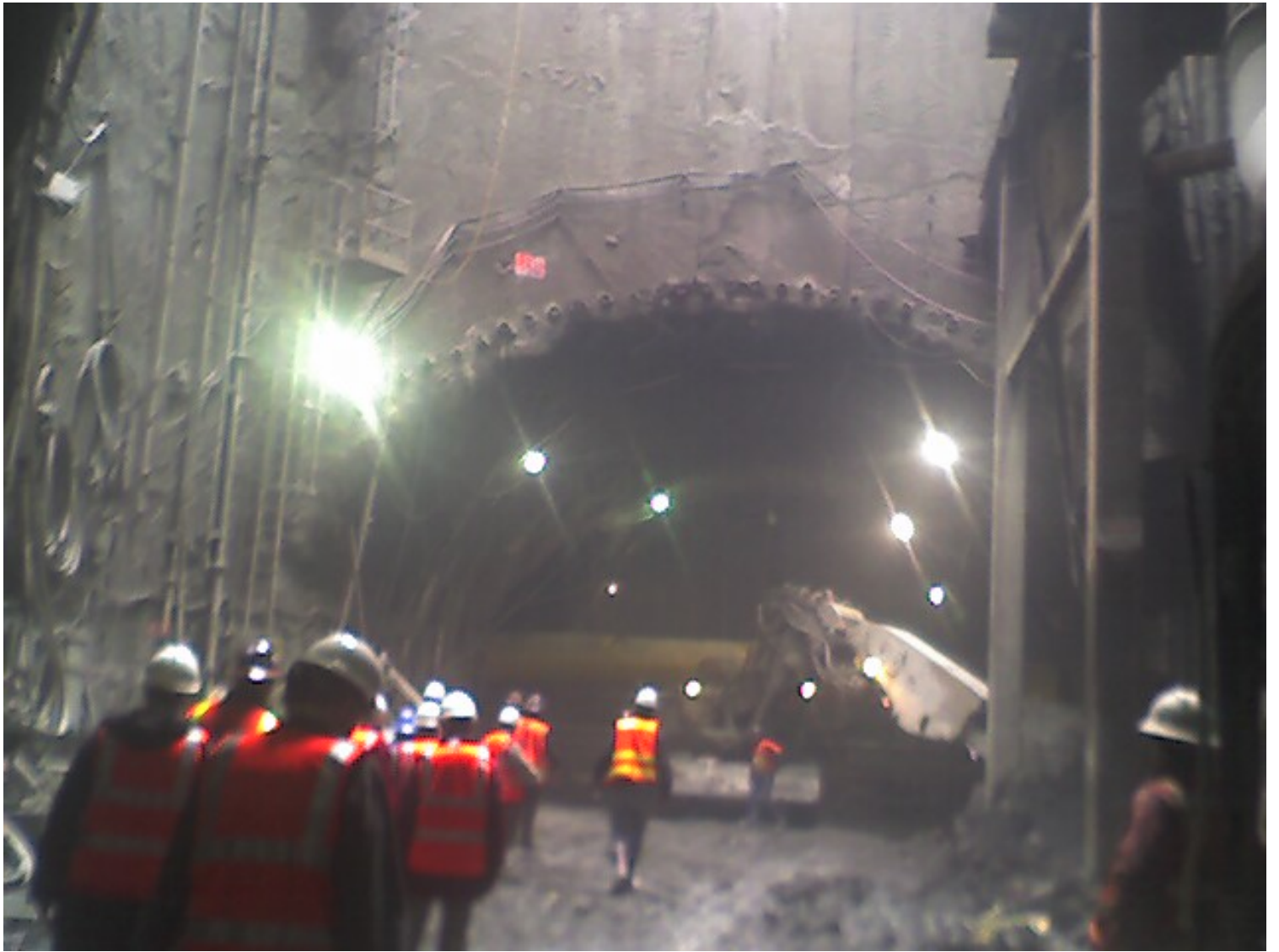
Beacon Hill tunnel work site
