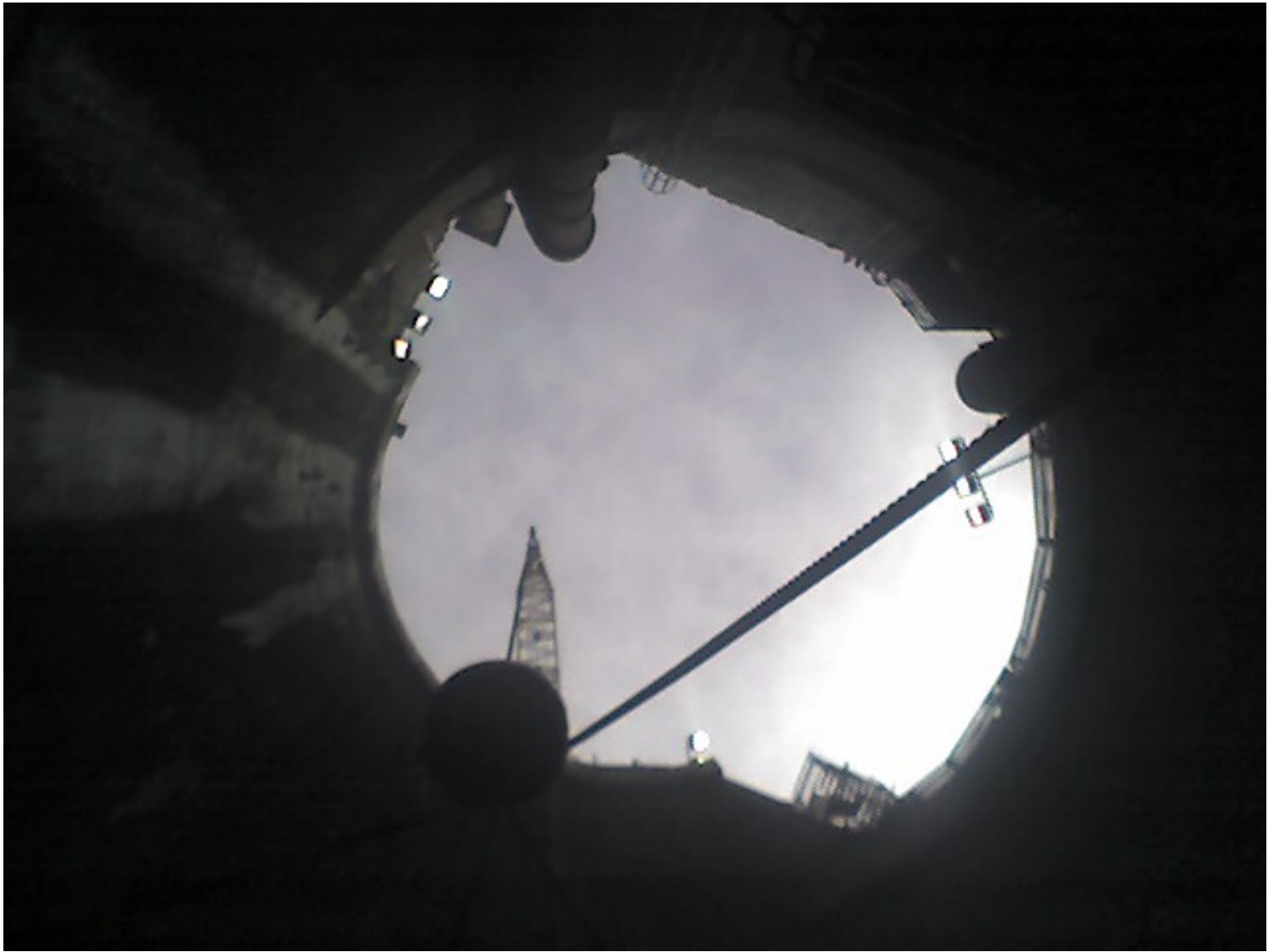
Looking up from Beacon Hill tunnel work site
