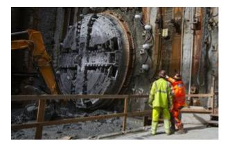
The cutterhead of the Northgate Link tunnel boring machine (TBM1) is brought out of a 95-foot-deep retrieval shaft at the University of Washington Station
