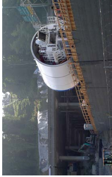
The tunnel boring machine is being prepared to dig through the side of Beacon Hill near Forest Street, under I-5, as part of Central Link light rail.
