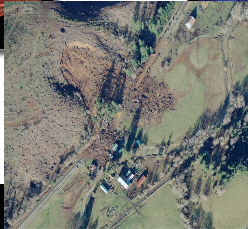
This is the aerial photo of the SR 6 Slide showing severe slide damage.
