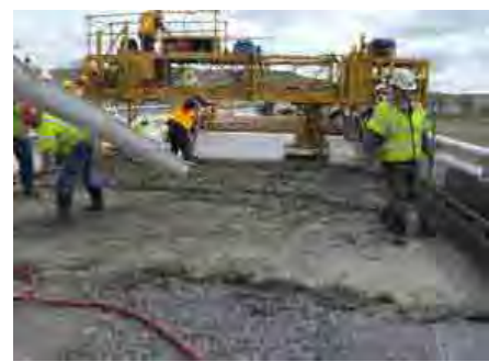
Pouring a 1.5 inch thick concrete overlay.
