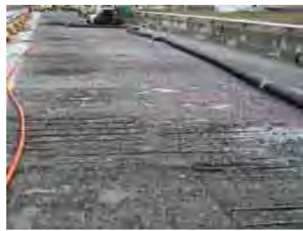
Deck prior to repair or overlay.
