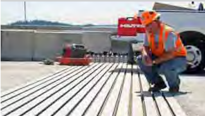
New expansion joint on the I-90 Homer Hadley Floating Bridge.
