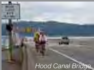
Hood Canal Bridge
