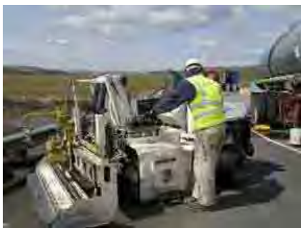
Hydro milling machine used to prepare the deck.
