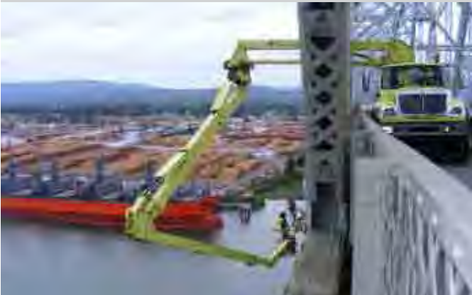
WSDOT bridge inspectors using a UBIT on the Lewis and Clark Bridge.
