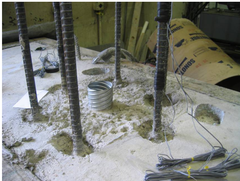
Figure 3-2. Specimen LB7-PT cap-beam after casting.
