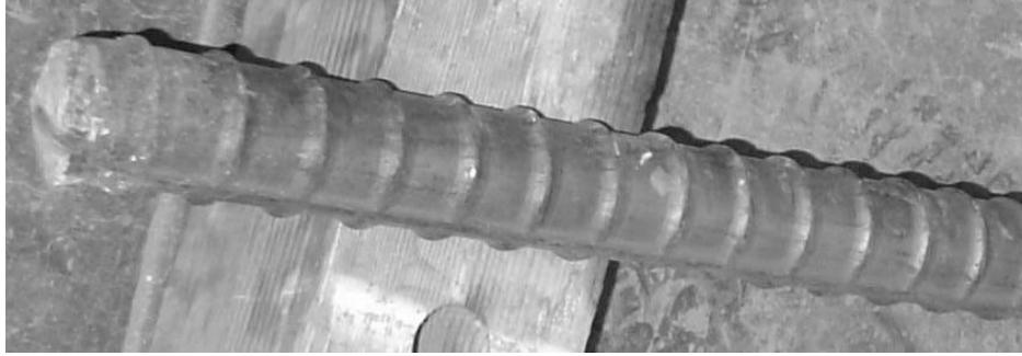
Figure 2.2: Bamboo ribs on a #18 bar
