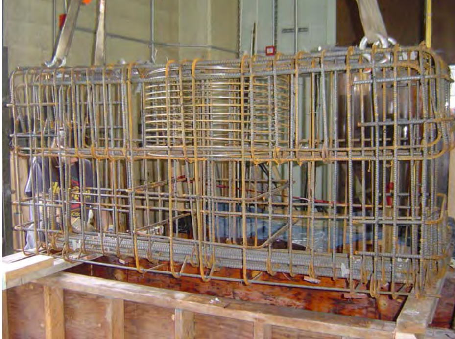
Figure B-27: Cap-beam and diaphragm reinforcement cage.
