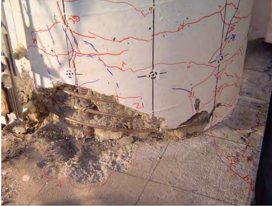
Figure 4-22: Spalling in the cap-beam and column in Specimen LB8-FB at Cycle 26 (2.92%/-2.85%)
