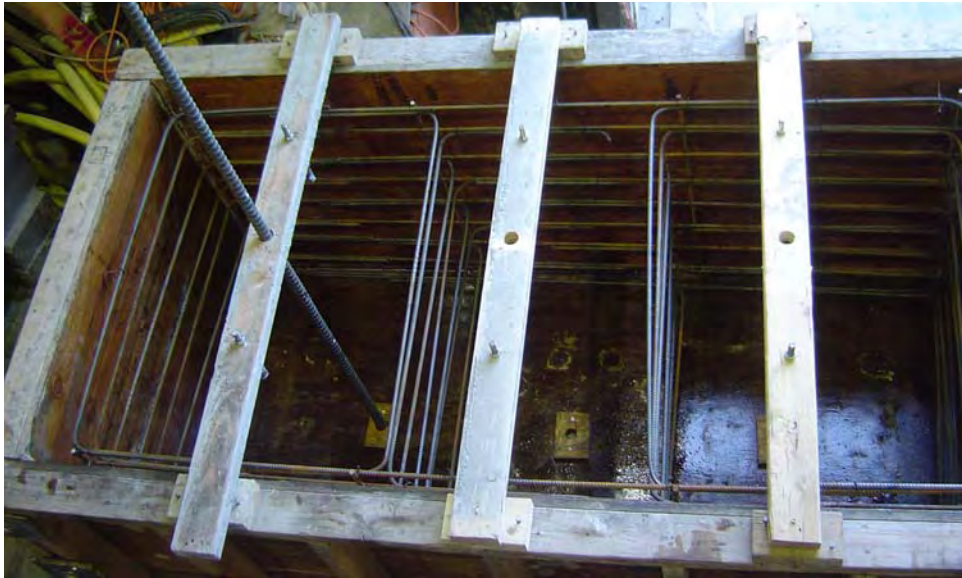
Figure D-3: Reinforcement and formwork for casting pullout specimens.
