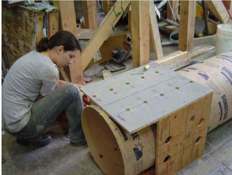
Figure B-36: Template used to cut holes in the Sonotube
