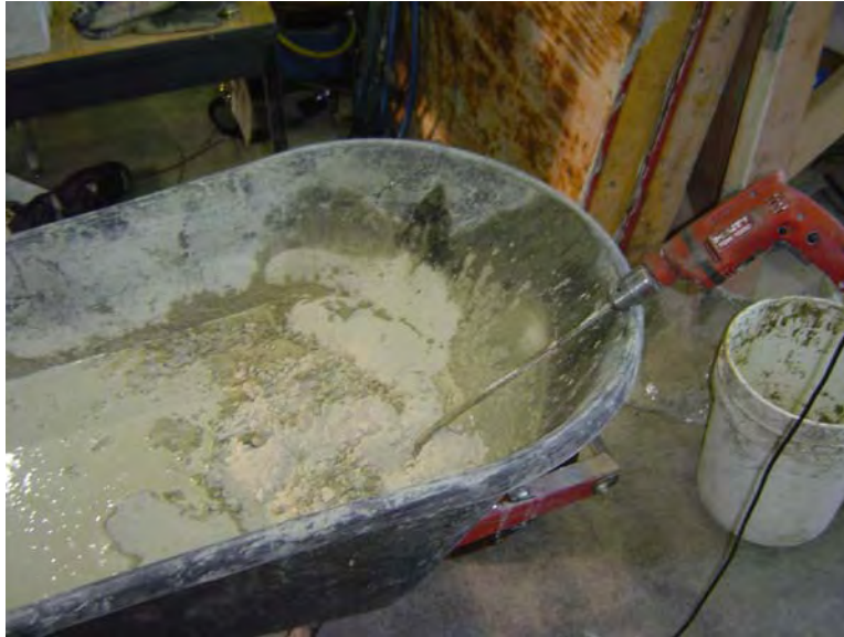
Figure B-14: Batching of grout mix
