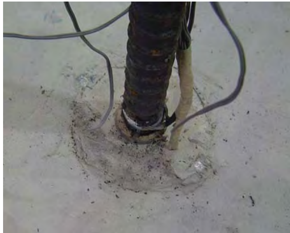
Figure D-11: No surface damage to Specimen AD8-D1
