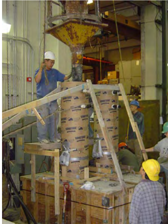
Figure B-38: Concrete placement in column using a bucket and tremie.
