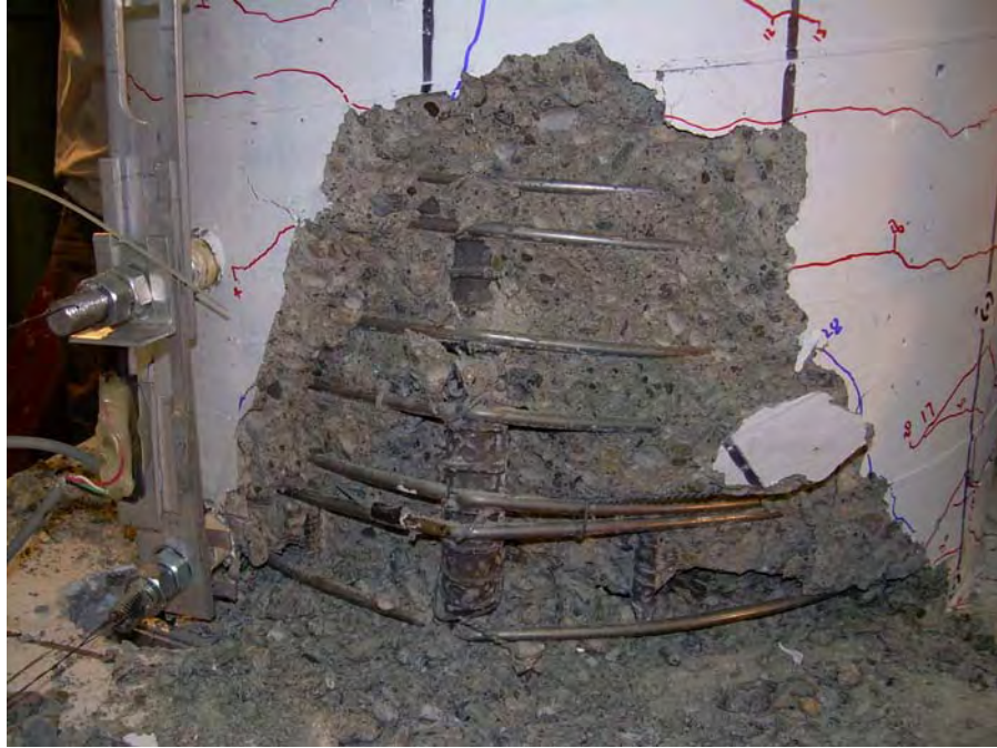
Figure 4-39: Bar 1 buckled and spirals fractured in Specimen LB8-D1 during Cycle 33 (7.11%/-6.93%)
