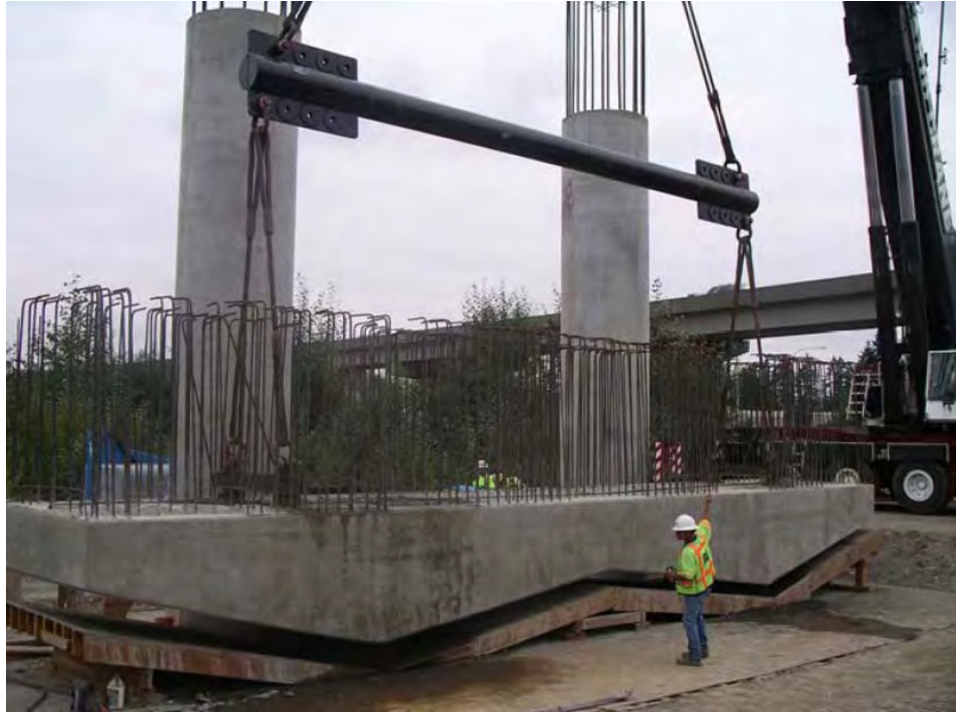
Figure 2-9: Lifting of the cap-beam from its forms (WSDOT 2007)
