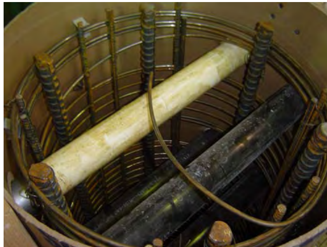
Figure B-37: Column formwork with PVC pipes installed
