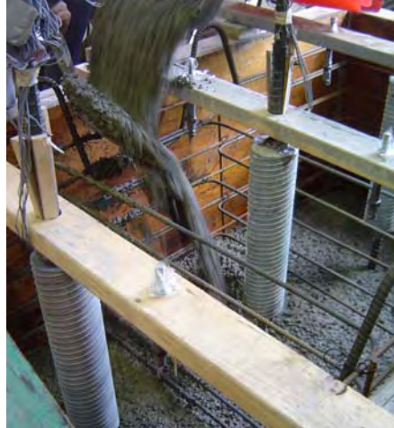
Figure D-4: Casting of the pullout test specimens
