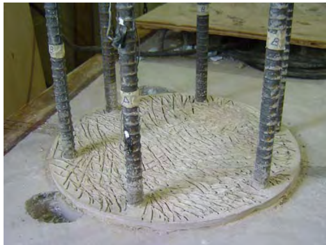
Figure B-33: 0.5-inch thick grout pad with raked finish
