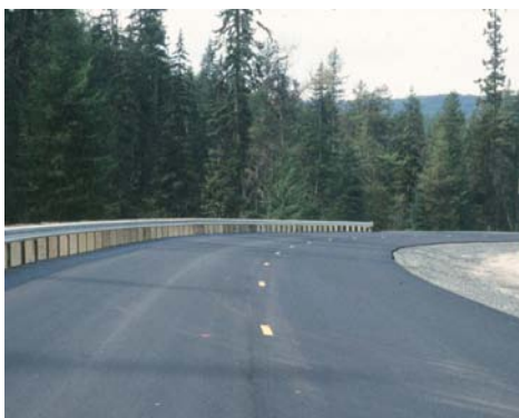
Photo 5. Final asphalt overlay on SR 20 with rock cap material in place.
