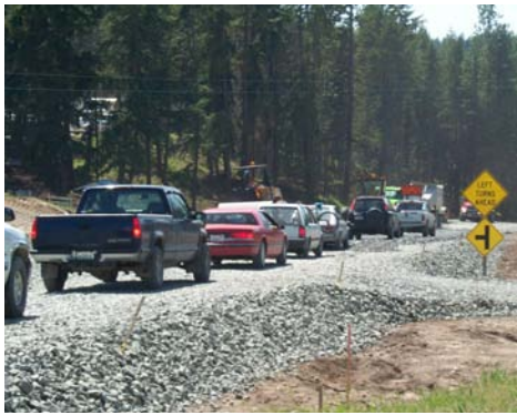
Photo 4. Vehicle traffic driving on the compacted rock cap surface.
