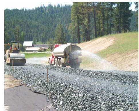
Photo 3. Watering and compaction of rock cap aggregate.
