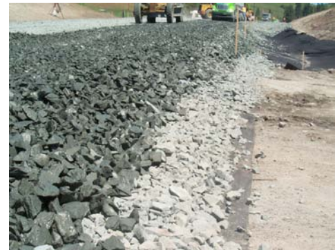
Photo 2. Open graded nature of the rock cap aggregate provides a positive drainage blanket allows excess water to be eliminated.
