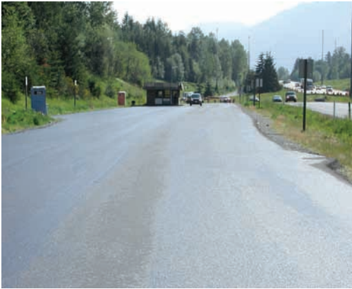
Completed pavement surface at a weigh station.
