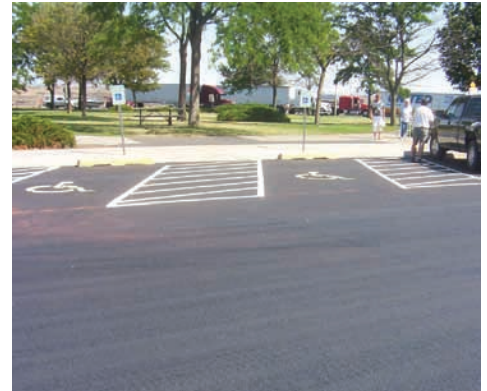
WSDOT rest area resurfaced with a sealer.
