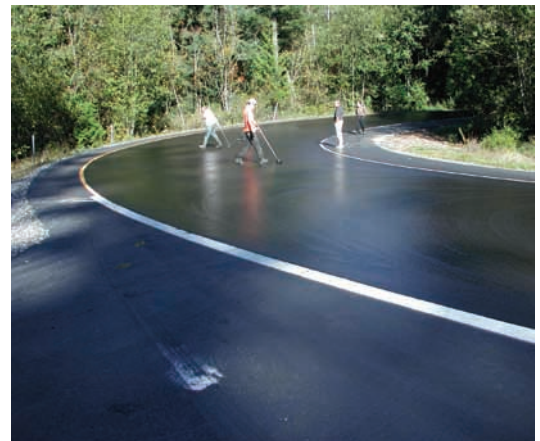
Hand finishing surface after final application of sealer.
