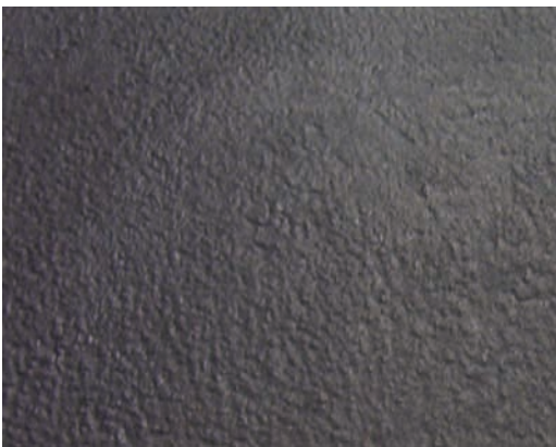
Completed pavement surface after sealing.
