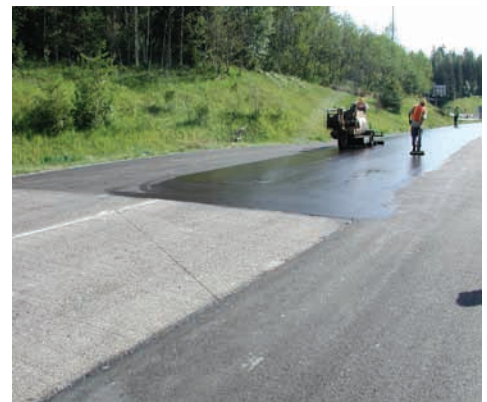
Sealer application applied at a weigh station.
