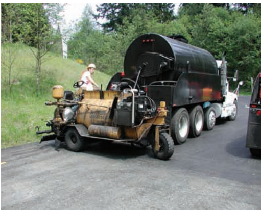
Resupplying a sealer application vehicle with sealant from delivery tanker.
