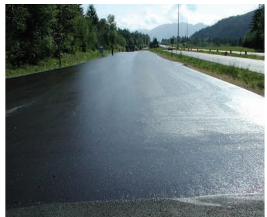
Completed surface prior to curing of sealer.
