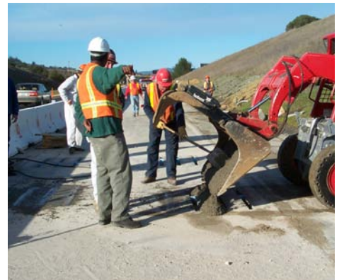
Photo 8. Placing grout in slot.
