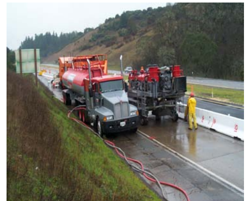
Photo 2. Slot cutting (gang saw).
