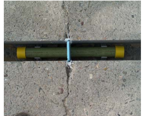
Photo 7. Dowel bar placement in slot.
