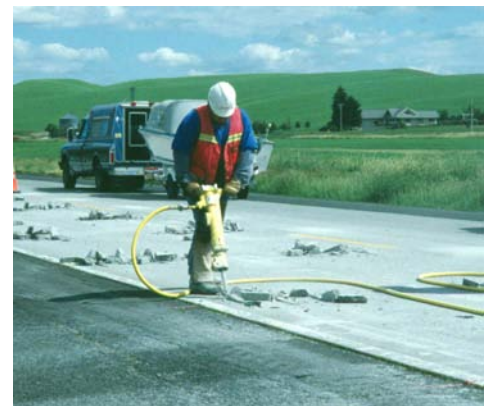
Photo 3. Removing slot.
