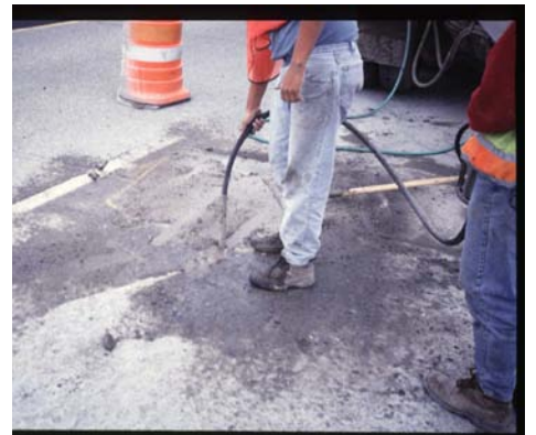
Photo 9. Consolidating grout in slot.
