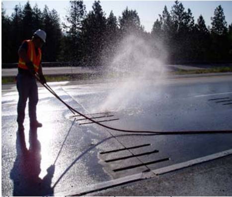
Photo 4. Slot cleaning with pressurized water.
