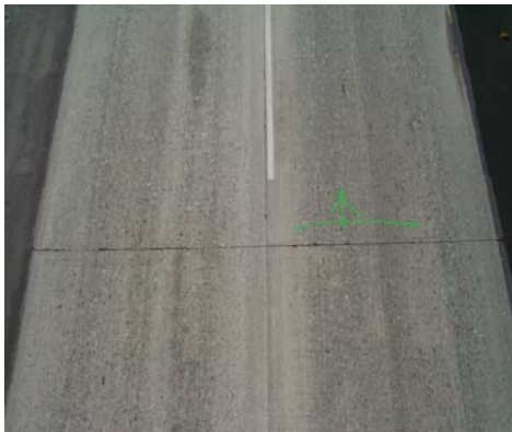
Photo 13. Retrofit lanes after grinding.
