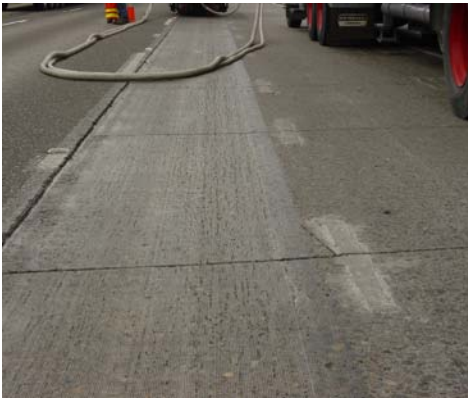
Photo 11. Grinding pavement after retrofit.
