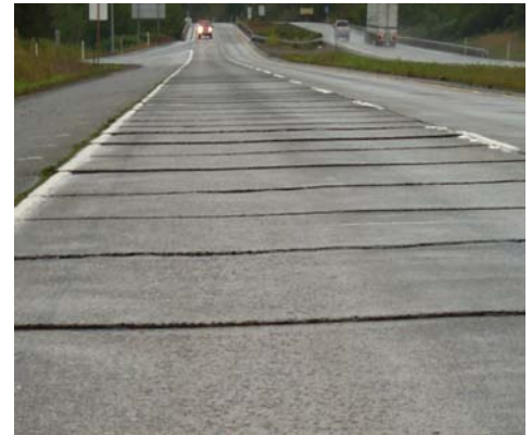
Photo 1. Joint faulting.
