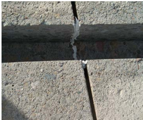
Photo 6. Caulking placement.
