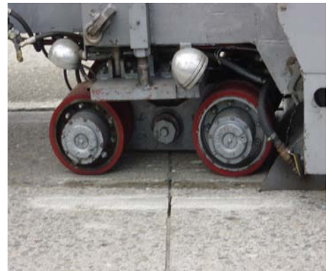
Photo 10. Grinding pavement after retrofit.
