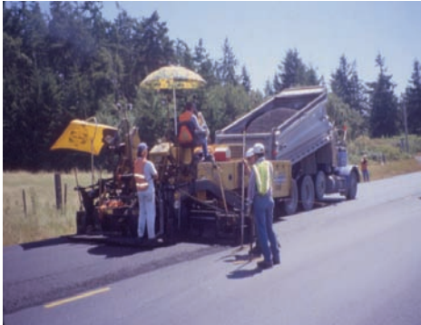
Image 3 - Dumping asphalt mix into the paver
