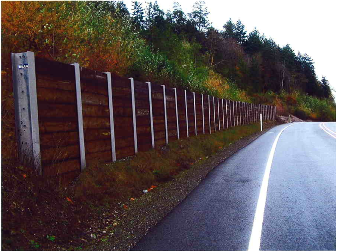
Figure 7. A photo of the soldier-pile wall option for containing debris flows.
