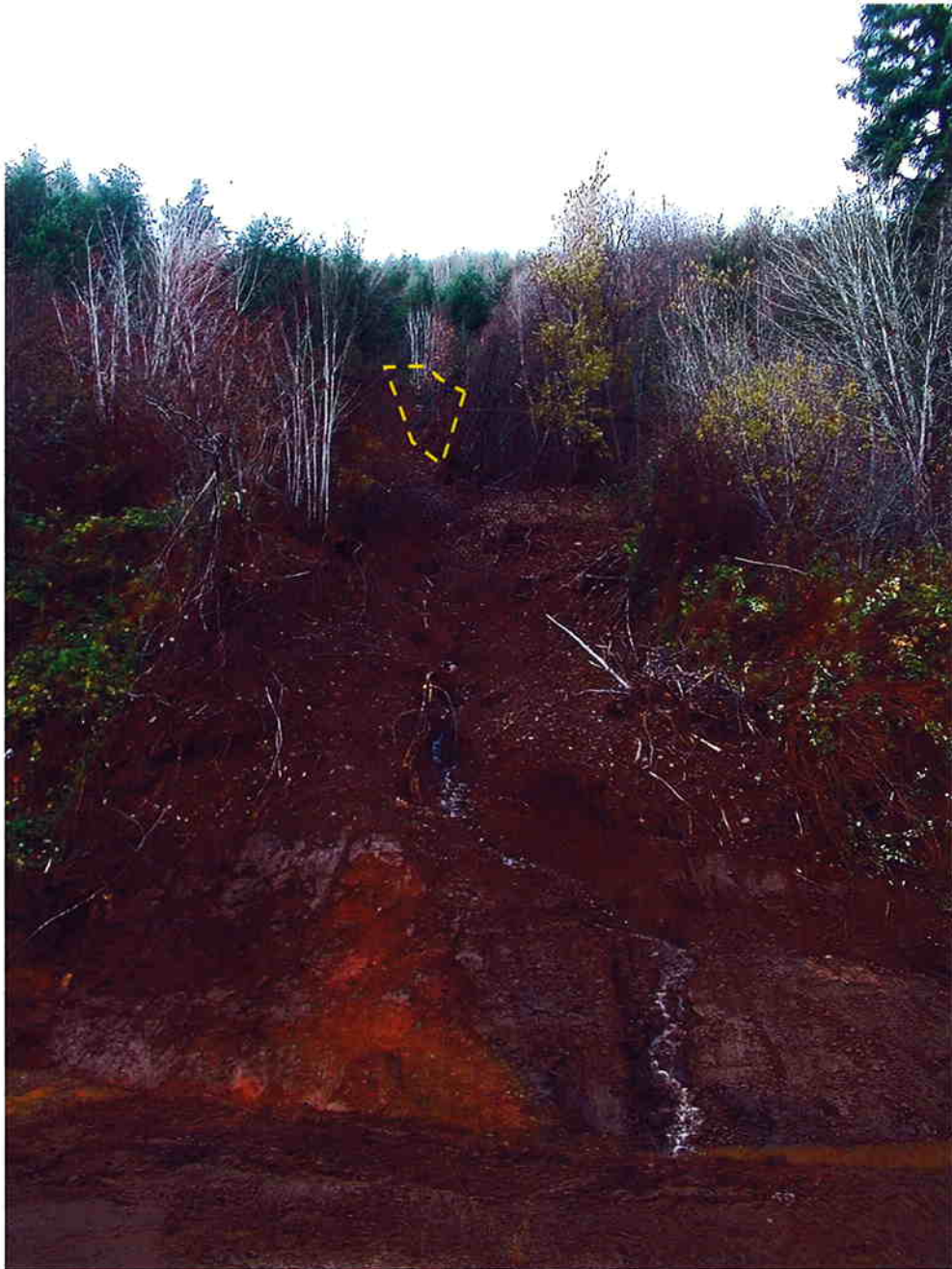
Figure 6. A photo taken from the highway looking up the debris flow chute on November 14, 2006 during road clean-up activities. We have approximated the area of the northern detached mass with a dashed, yellow polygon.
