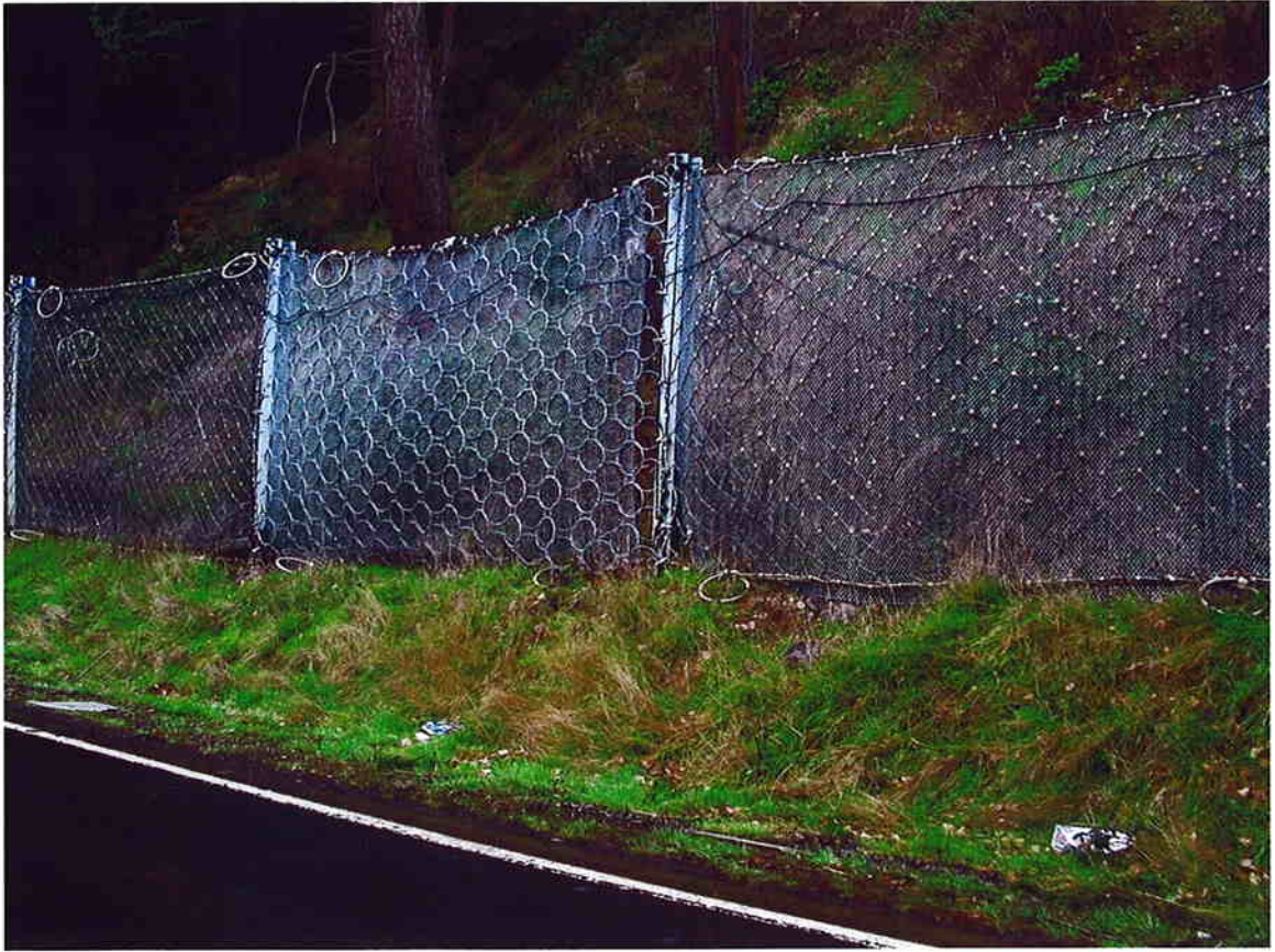
Figure 8. A photo of a typical debris flow fence constructed on SR 4.
