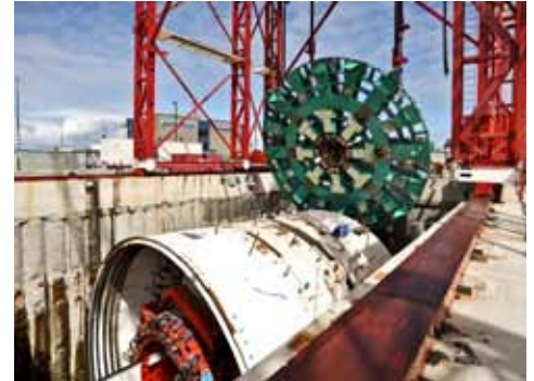
Bertha's massive cutterhead being carefully lowered into the 80-foot-deep pit.
