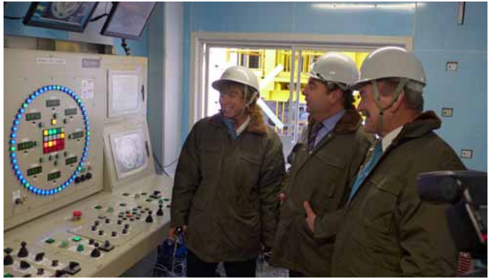
Inside the control room of the tunneling machine.
