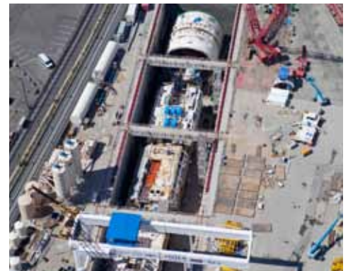
Aerial view of the SR 99 tunneling machine and launch pit.
