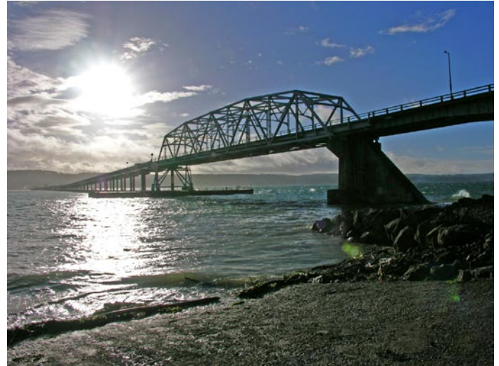
The Hood Canal Bridge serves as a vital economic and social link between the greater Puget Sound and the Olympic Peninsula.
