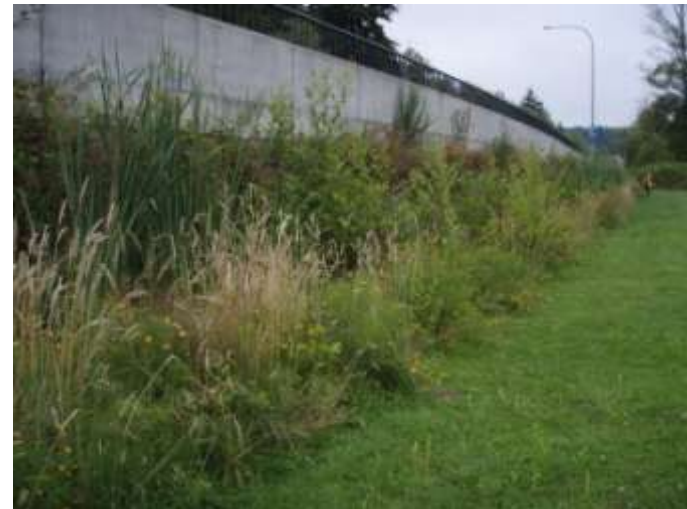
Photo 3 Woody cover at Wall 10 (July 2010)
