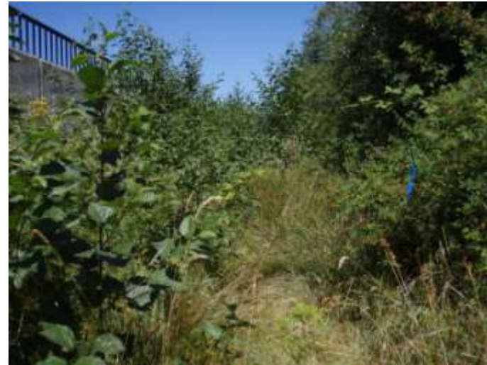
Photo 1 Invasive cover in temporarily impacted retaining wall area (July 2010)
