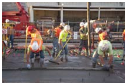
K-G crews work on the project's final pontoon pour. June 27, 2008.
