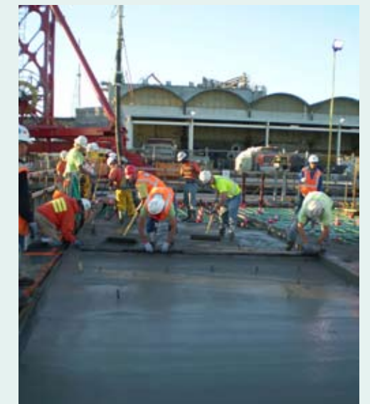
Crews at CTC start work on the final pontoon pour of the project. June 27, 2008.
