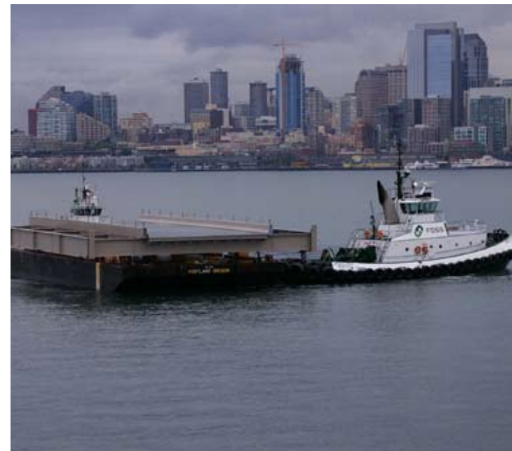
(left) The first of three lift spans completes its 358-mile trip from Vancouver, Wash. to Seattle. June 9, 2008. (right) The second and third lift spans are towed into Seattle. June 23, 2008.
