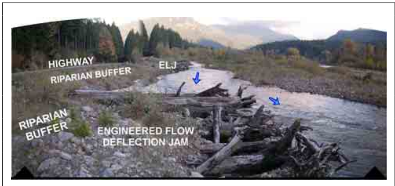
Figure E-17. View of ELJ flow deflectors in the Cispus River, (shown in Figure E-16) 1 year after installation. Note the establishment of the riparian buffer along the highway.
