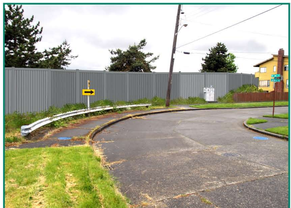
Preliminary design concept showing Tuf-Barrier or Carsonite at NE 81st Street and Latona Avenue NE looking west
