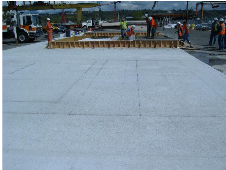
Workers prepare a casting bed for the concrete pour, April 18, 2007.
