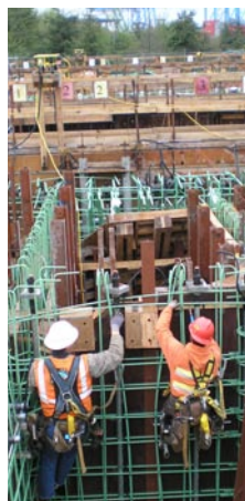
Carpenters install box girder blockouts on pontoon NA, April 25, 2007.
