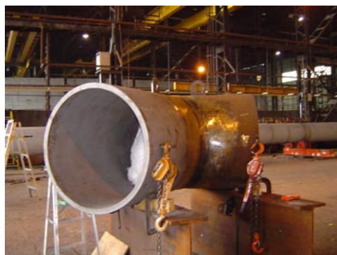
Crews complete a mockup for the welding of the transition spans, September 7, 2007.
