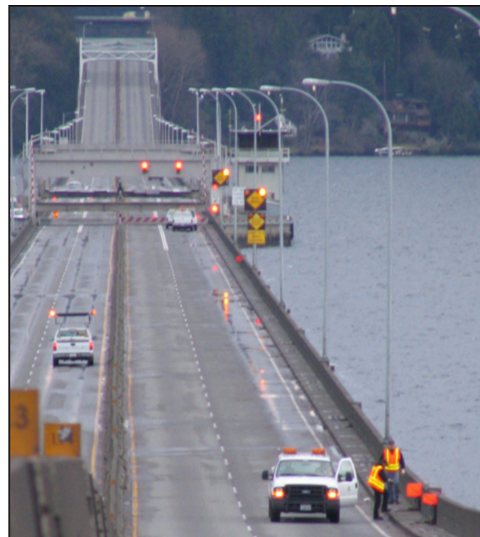
SR 520 bridge closed for inspection
