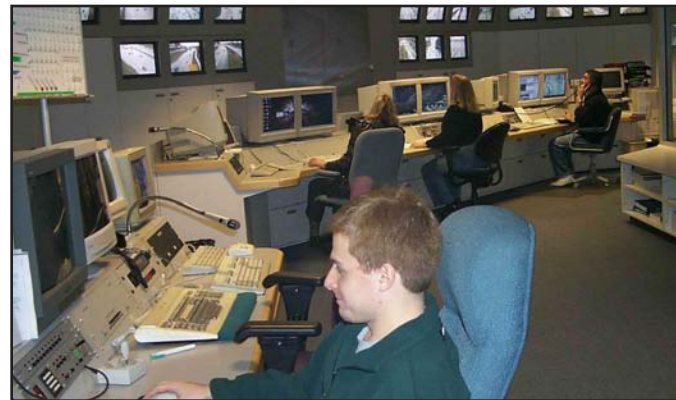
WSDOT's traffic management center in Shoreline
