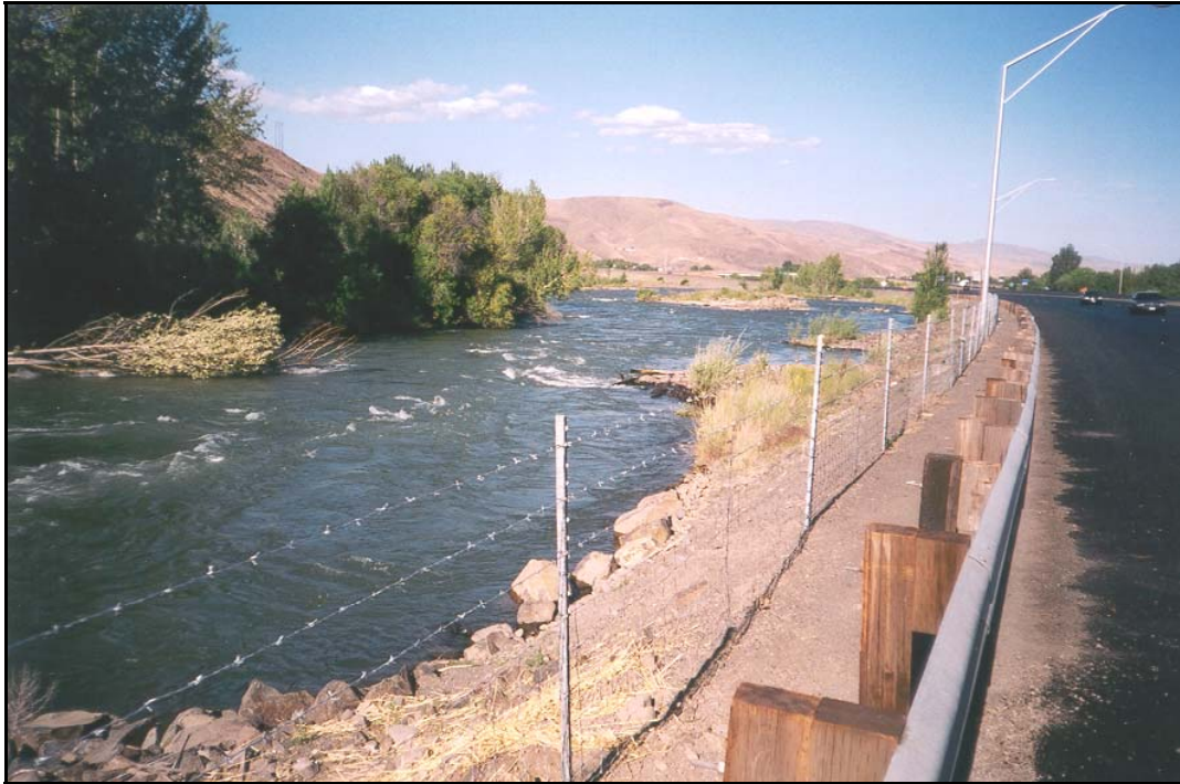
Figure 2: Photograph taken from westbound side of US 12, approximately 3,000 feet upstream of 16 th Avenue. Note rock at toe of highway prism and groins and barbs extending into channel.
