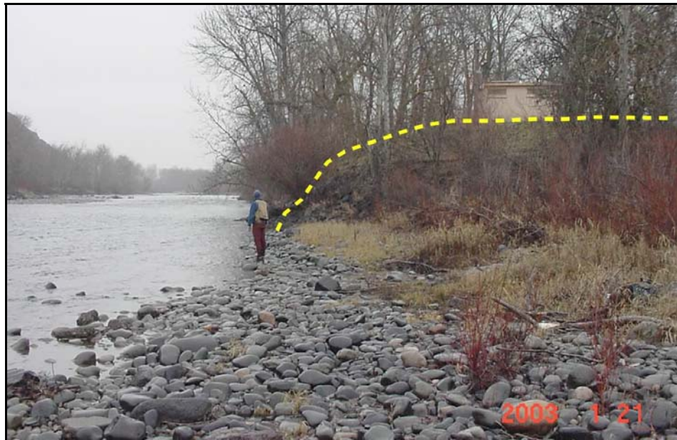
Figure 4: Floodplain and perhaps a portion of the active channel have been filled for the City of Yakima's Ranney-type diversion structure and pump located near Station 16000. Yellow line in figure highlights the extent of fill, which is over 20 feet above the riverbed.
