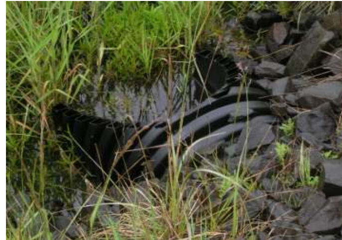
Photo 1 Flow observed in the culvert under North Fork Road (June 2010)
