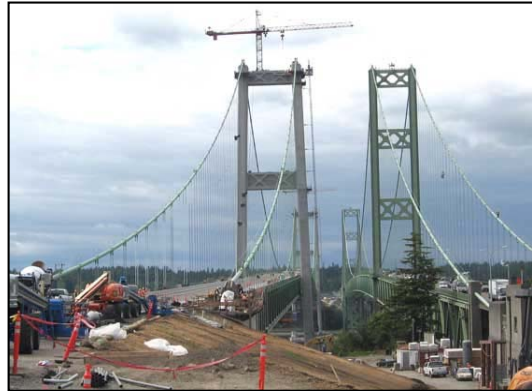
Tacoma Narrows Bridge construction.
