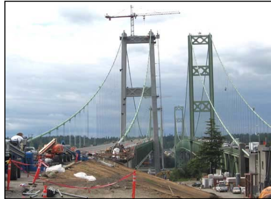
Tacoma Narrows Bridge construction.
