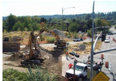
Drainage Work on SE 8th Ramp.
