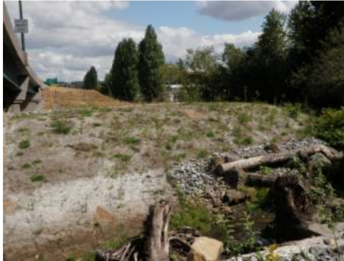
Photo 3-Bank logs in Springbrook Creek (July 2010)
