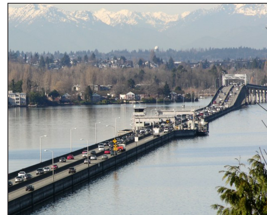
Traffic on the existing SR 520 floating bridge
