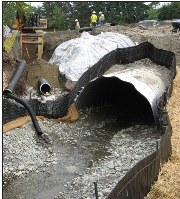
New and wider culverts will provide better fish passage on the Eastside.
