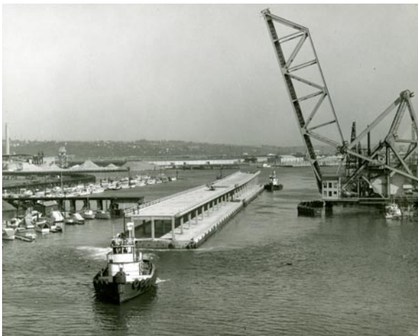
The first Hood Canal Bridge pontoons are floated out of Tacoma in 1960.
