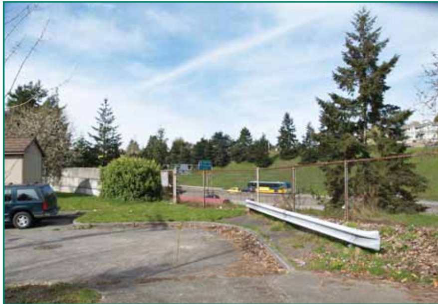
Existing conditions at NE 77th Street looking northeast
